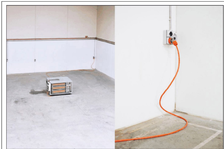
Fig 1. The Relectrify energy storage system in Melbourne on Jan. 17
